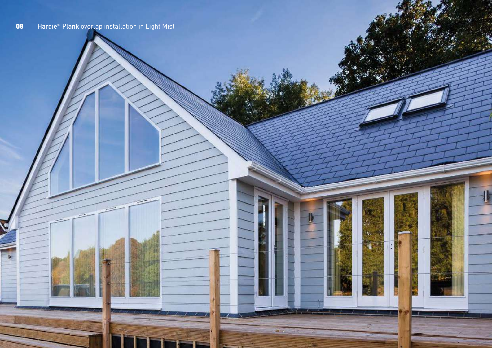
Hardie® VL Plank horizontal installation in Light Mist
